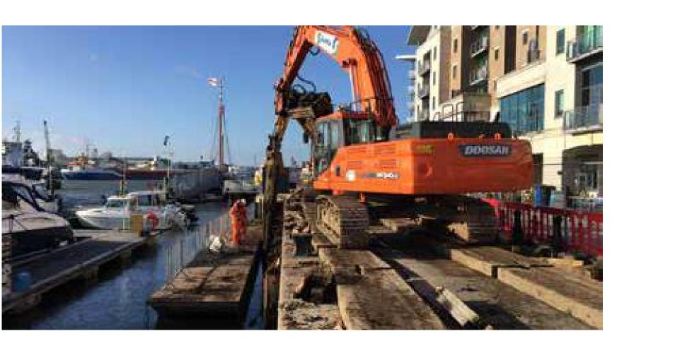
An example of the construction methods used on Poole Quay for sea wall raising. The techniques will be similar along Back Water Channel. Zone A & C works will take place from the land but the vast majority of Zone E works will take place from the water.
