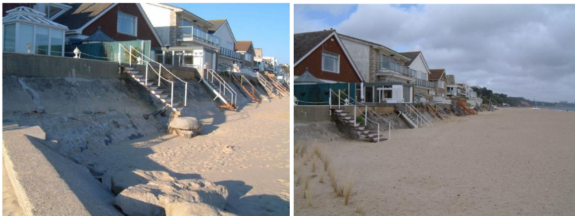
Figure 8 Before (left) and after (right) beach replenishment was carried out at Sandbanks in 2003, showing a large elevation in beach level (Robson, 2003).
