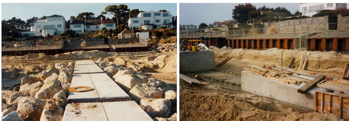
Figure 6 The construction of concrete walkways on groyne structures installed at Sandbanks.
