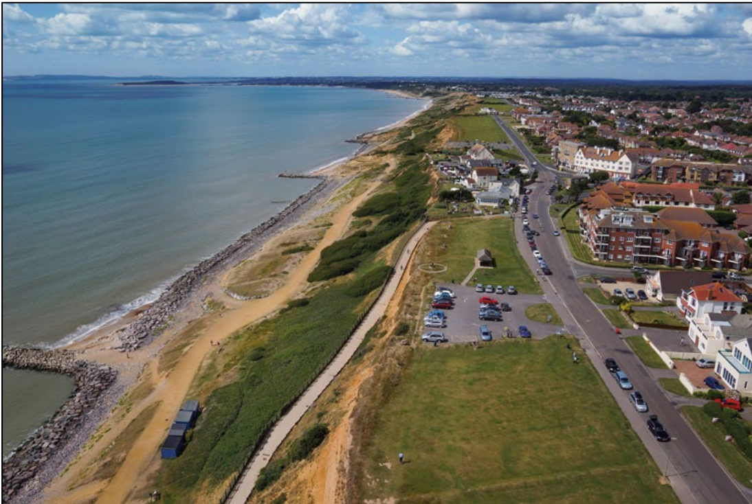
Aerial view looking west. (Source: Courtesy of Adrian Charters (QuarryDesign) and New Forest District Council).
